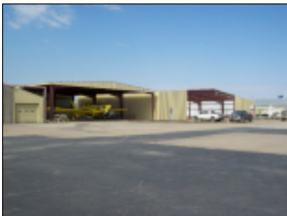
Framing up, metal going on
